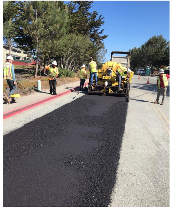
Trench restoration paving on Abrams
