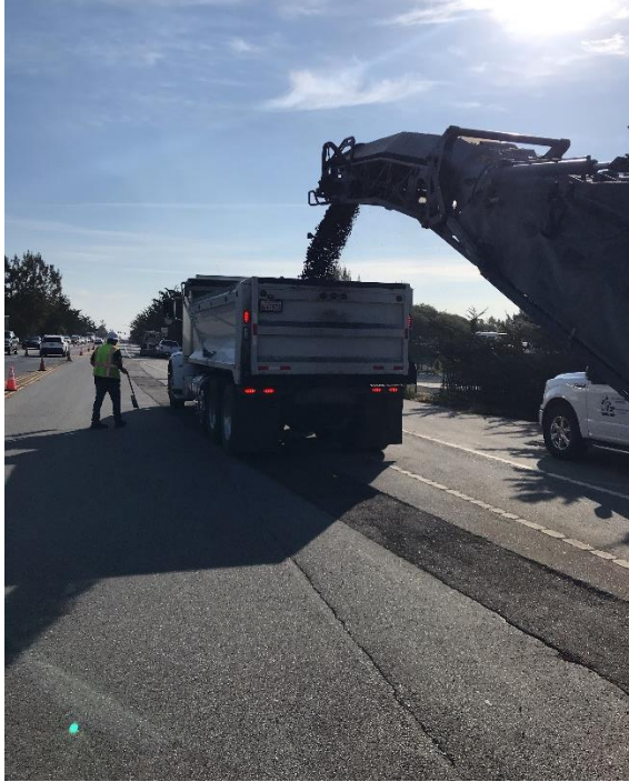
Grinding for trench restoration on Imjin Pkwy.
